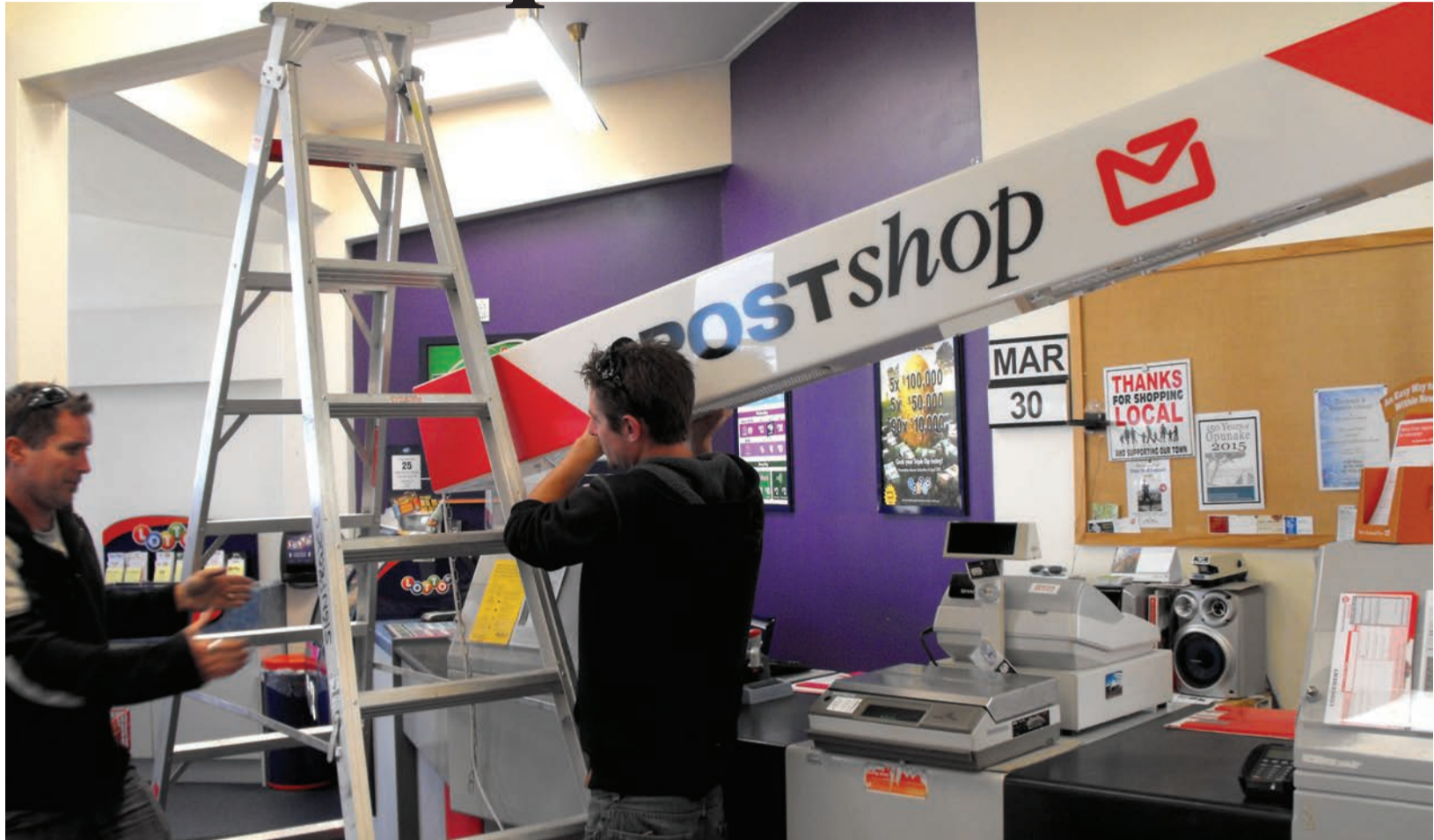
Dismantling our post office
